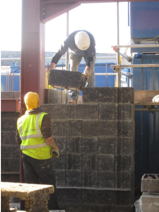
Durisol wall construction: The Hayridge
